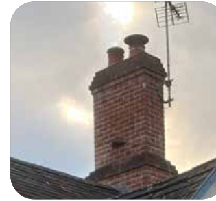
Tall decorative chimneys
