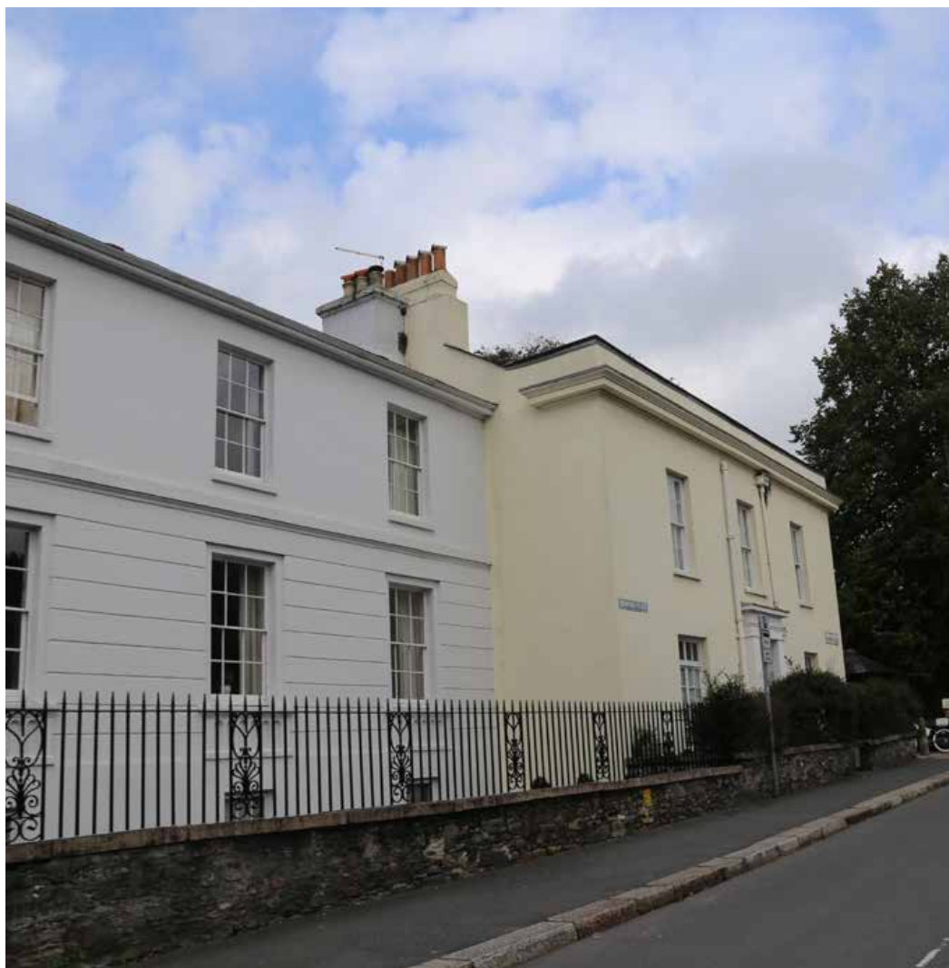
Figure 82: - Granite kerbs, stone wall with capping and railings. Building facades with generous windows and positive fenestration rhythm. Texture and subtlety with string course, plaster work and render detail all in white.
