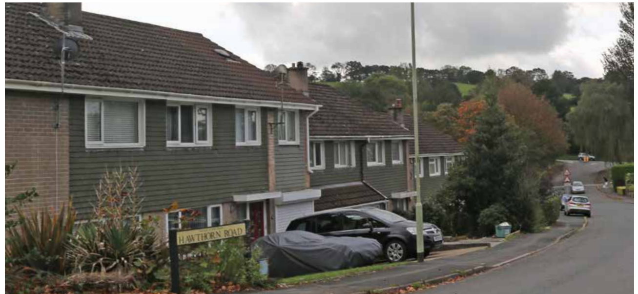
Figure 22: - Tiled panels are likely not cavity constructed and have minimal insulation and therefore more susceptible to elevated heat loss.
