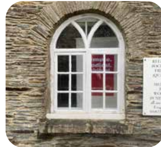
Varied stone arch lintels
