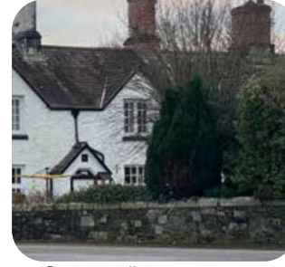
Stone wall, granite coping
