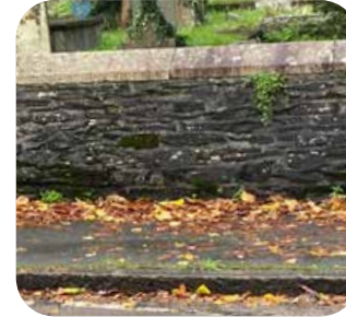
Stone wall granite coping
