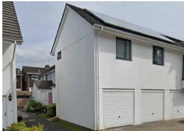
Figure 47: - Flats over garages. PV array on roof.
