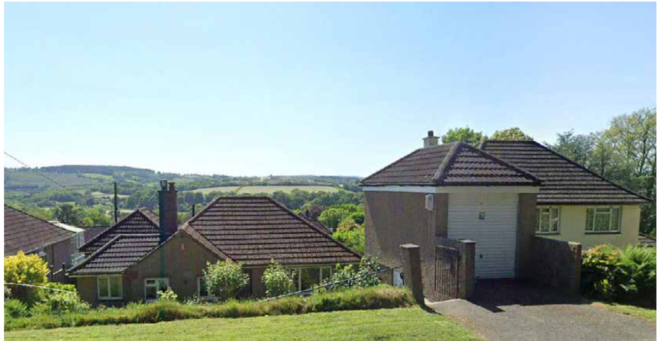
Figure 50: - Response to levels, Whitchurch Road.
