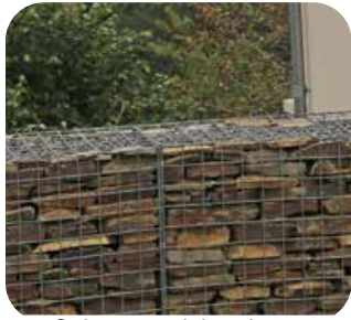
Gabions with local stone
