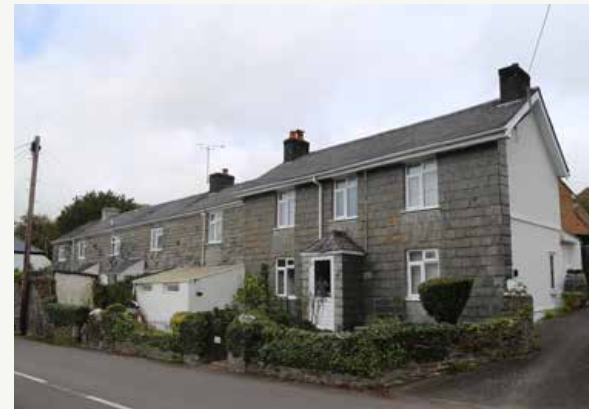
Figure 64: - Example short row terrace, which demonstrates the maximum single development size. Also a good example of slate hanging on the primary elevation.
