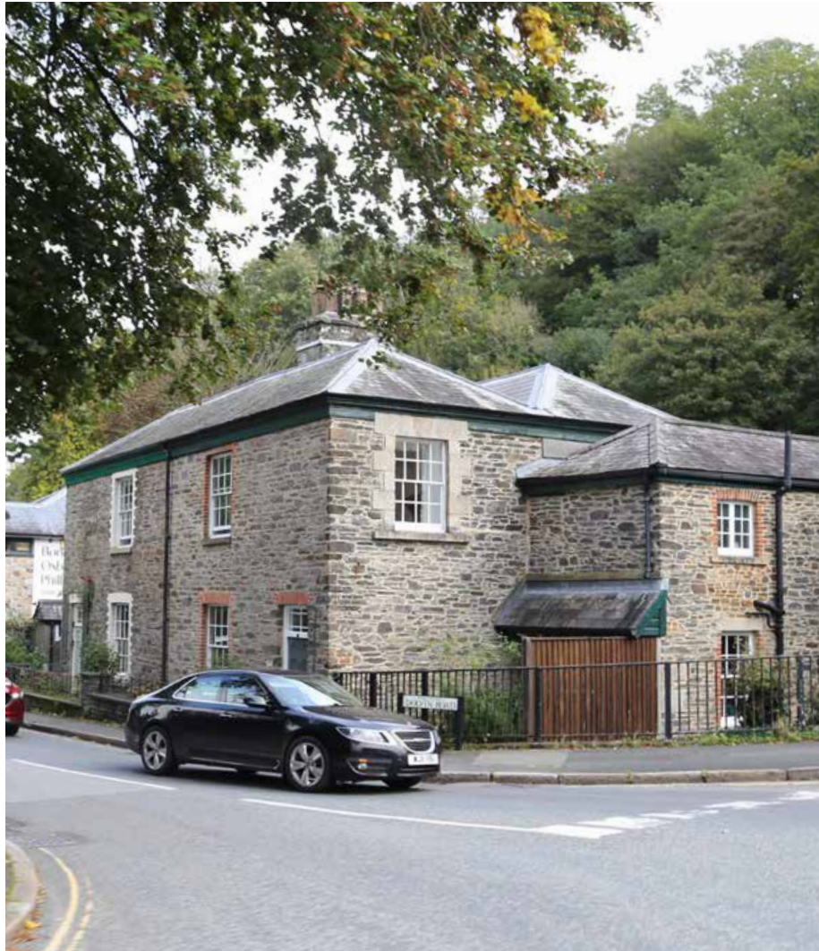
Figure 83: - Example of how stone could be used as a gateway development building. Note the use of granite lintel/surrounds and brick.
