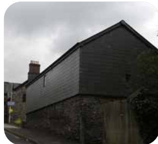
Slate hung upper storey
