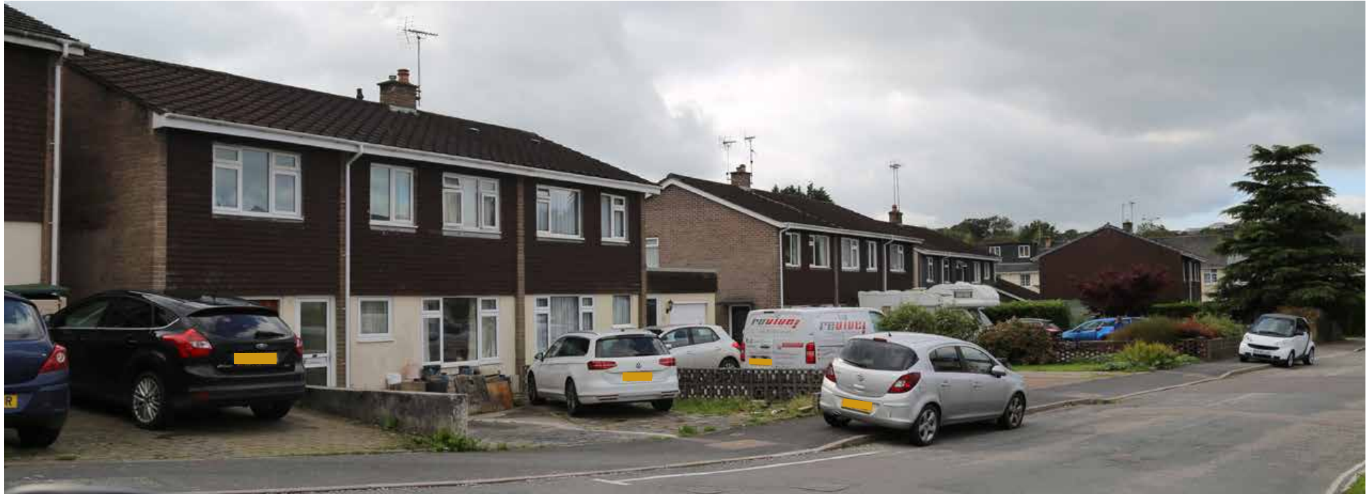
Figure 46: - Light coloured brick, render and concrete tiles, Grenville Drive.
