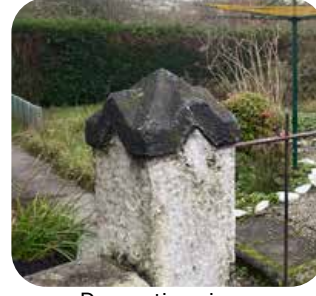
Decorative pier cap
