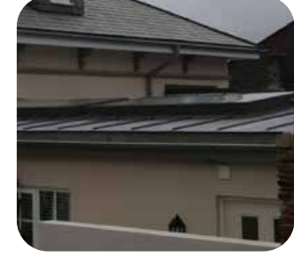
Standing seam with roof light extension roof
