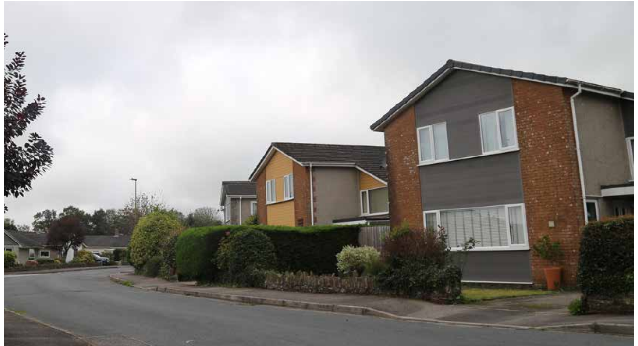
Figure 36: - Examples of material palette. Brown brick, concrete roof, roughcast render and recent composite cladding.
