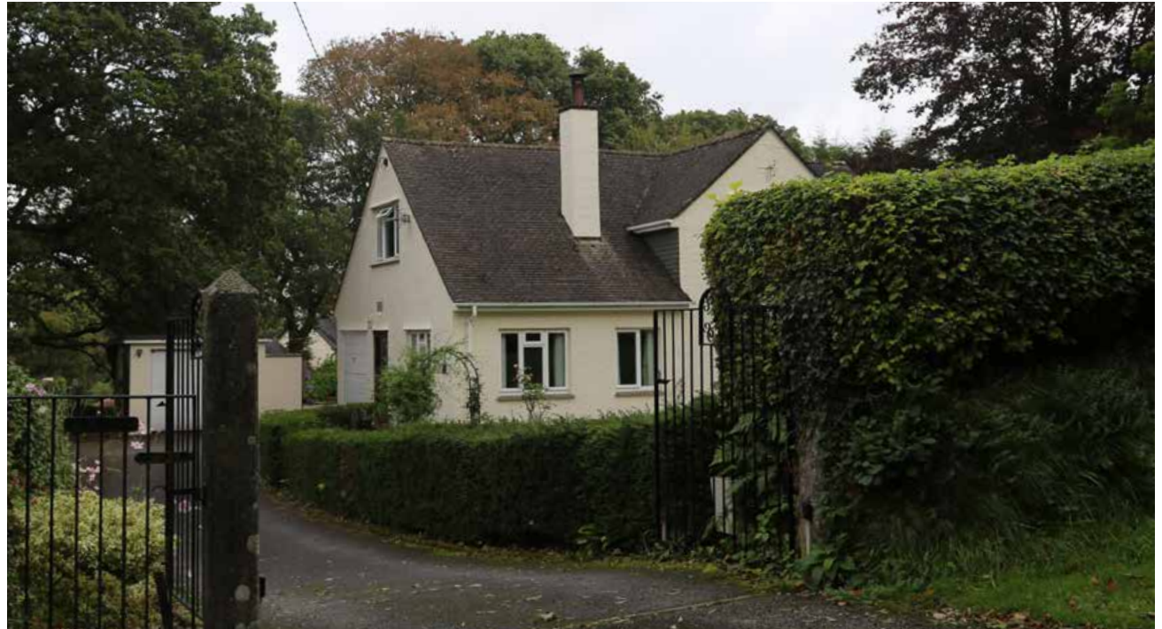
Figure 56: - Storey- and-a-half/two storey typology. Sympathetic concrete tile similar to slate.
