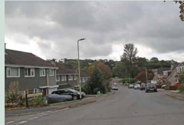
Figure 77: - Plot left susceptible to street water run-off.
