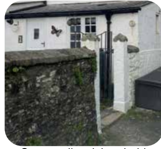
Stone wall and threshold
