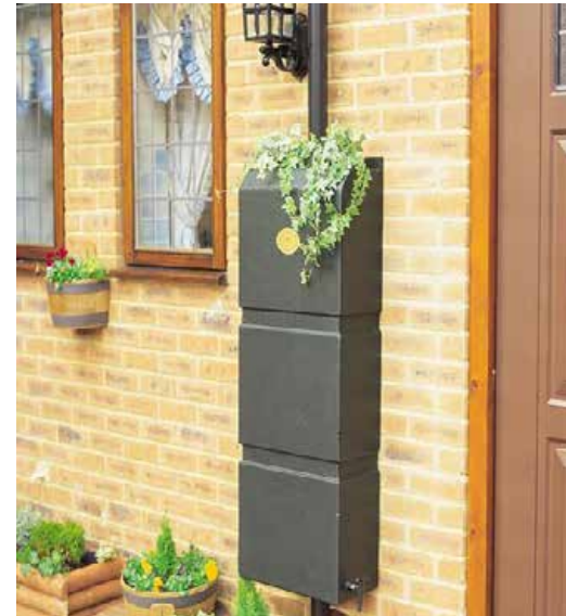
Figure 95: Example of a gravity fed rainwater system for flushing a downstairs toilet or for irrigation.
