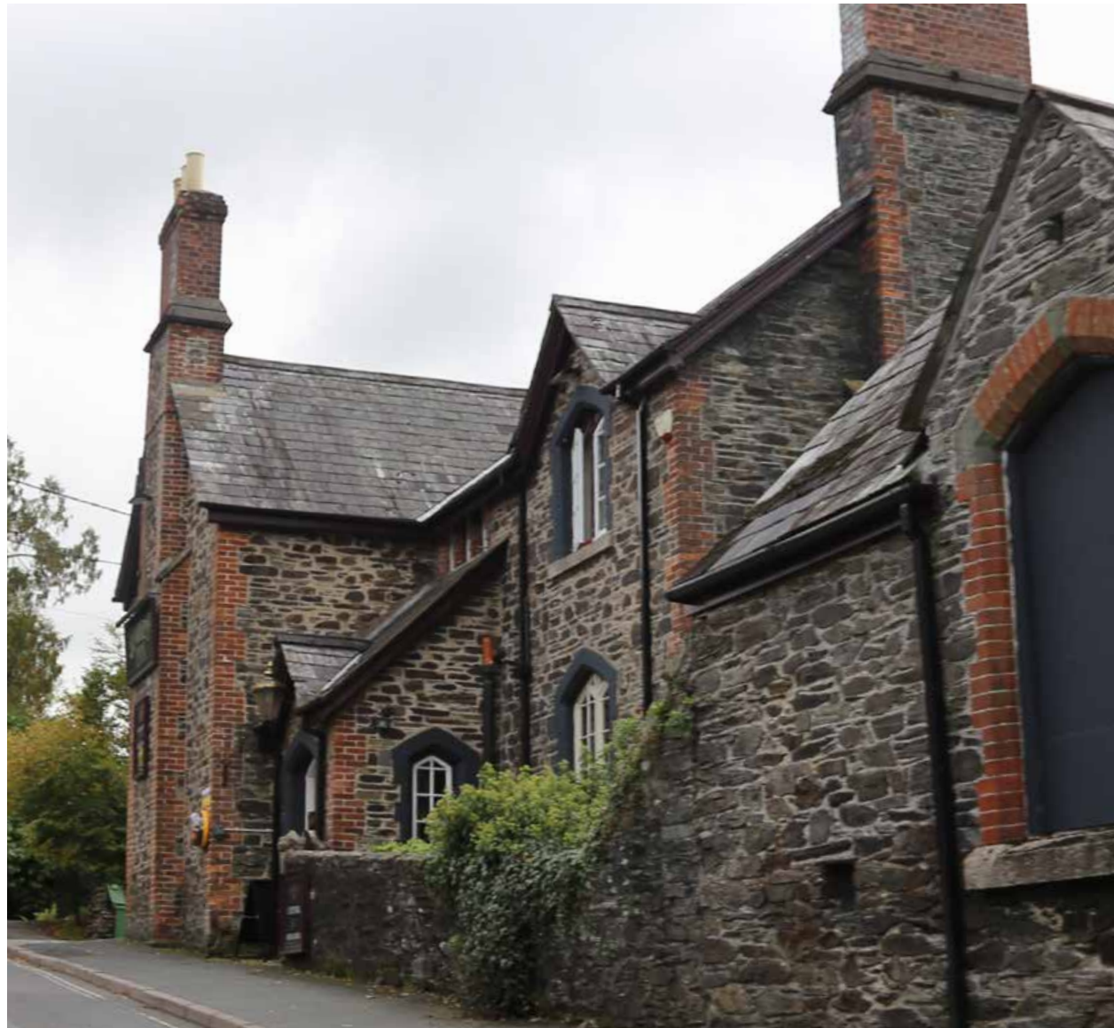
Figure 15: Market Inn, upright building construction in rubble stone with brick quoins and roofed in slate.
